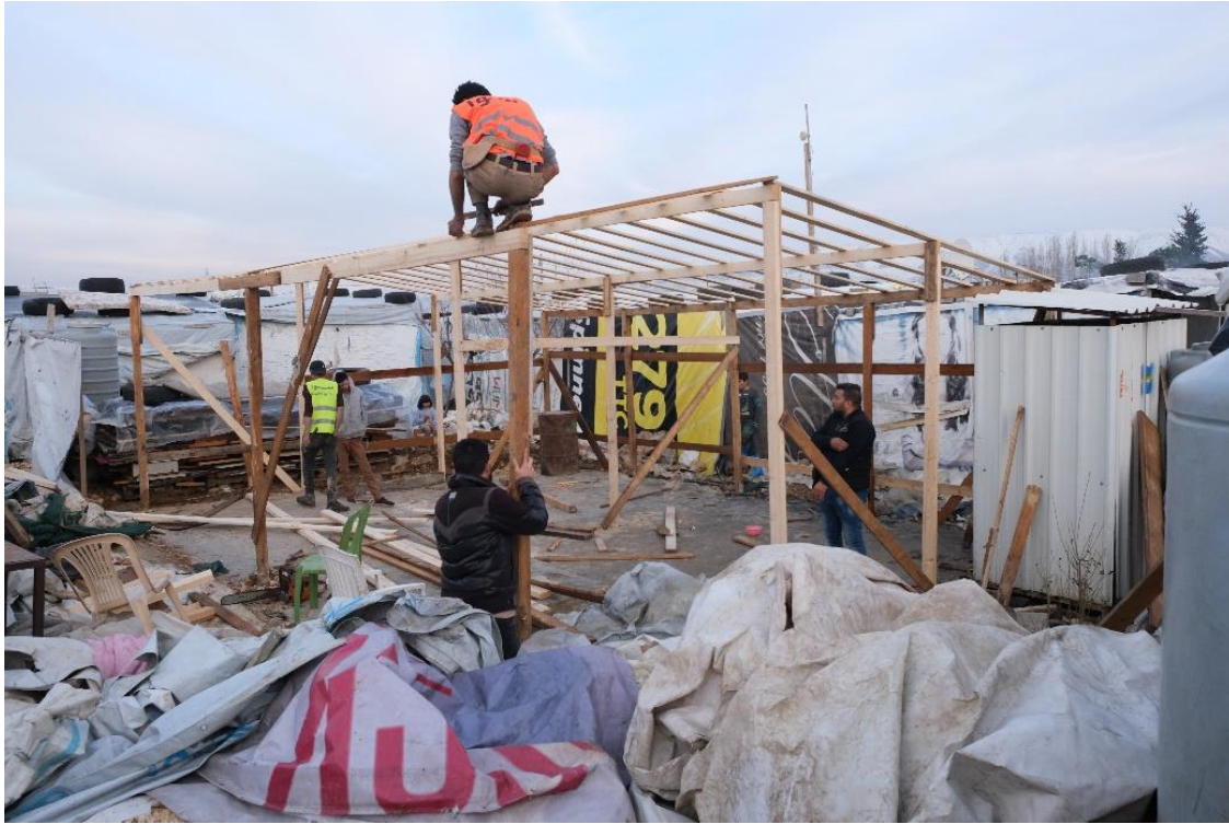
Pic9: Saadnayeel- SAWA's team with volunteers from the community during rebuilding damaged tents by using woods, shaders and many other materials provided in this project.
