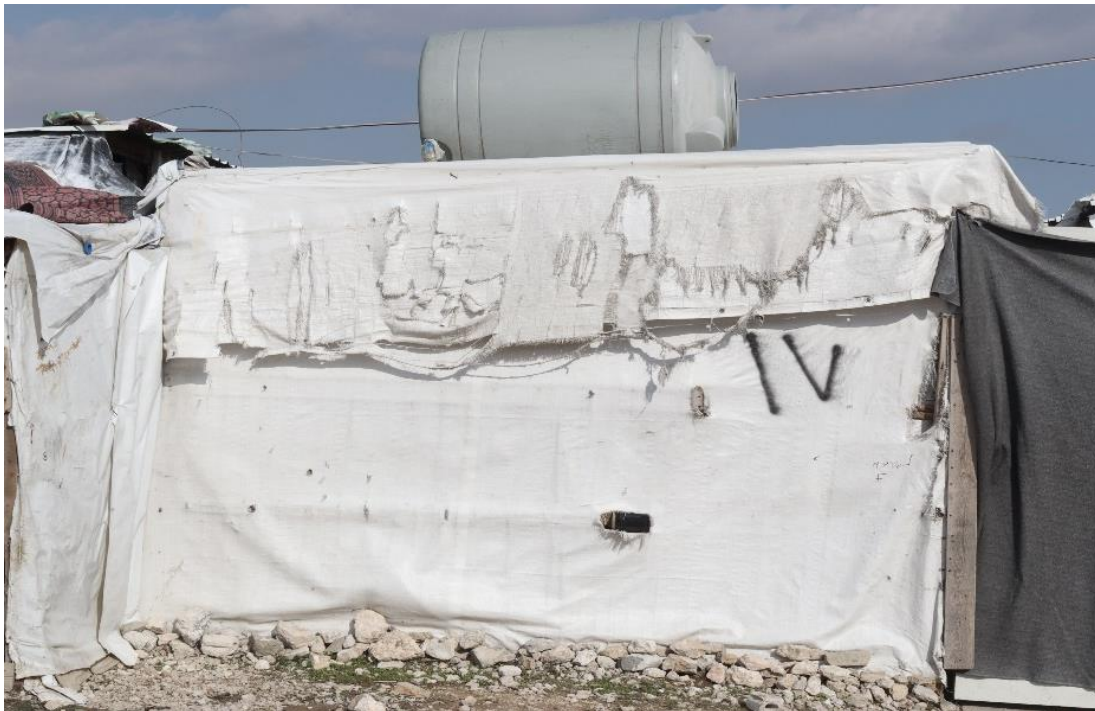
Pic4: Tent Shader for a damaged tent before providing new tarpaulin in Barlias camp
